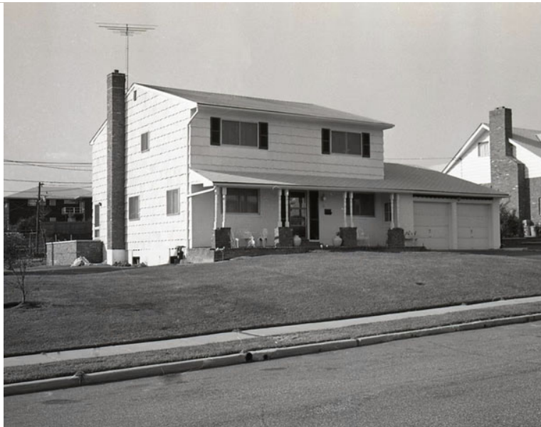
View from the street of the Franzese home on Shrub Hollow Road in Roslyn in November 1965. Photo credit: Marvin Sussman / Newsday
